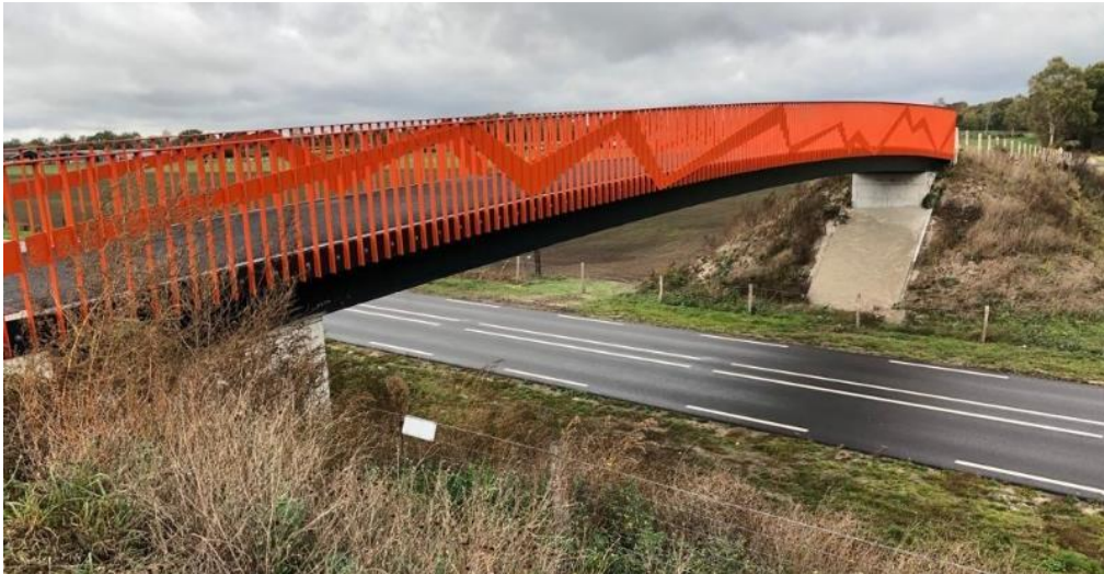
Composite footbridge in-situ, image courtesy FiberCore Europe: www.fibercore-europe.com/en/
